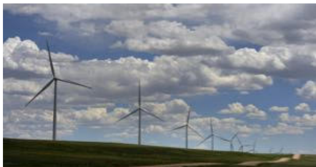
WIND TURBINES ALONG A RURAL COLORADO ROAD (Helen H. Richardson, The Denver Post,
