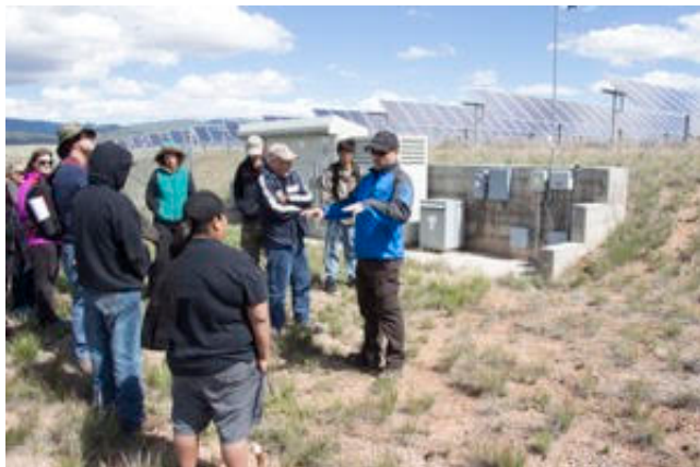
Dan Weinman, CEO of PPC Solar in Taos explains operations of the 500-kilowatt (kW) solar tracking array that powers the UNM-Taos Klauer Campus.
