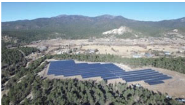
Picuris Pueblo Solar Photovoltaic (PV) Array, (Picuris Solar Farm), Vadito, NM.
